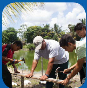
Trio School pond restoration project
